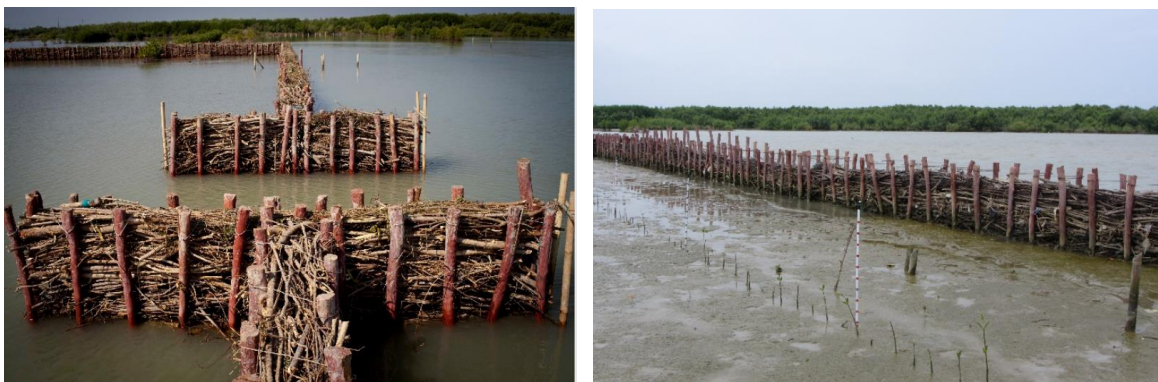
Figure 4: Sediment collection system for mangrove growth
